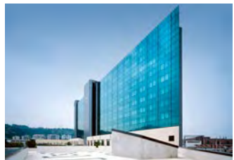
SHERATON HOTEL Genoa, Italy / 1993 Arch. Corradini, Serapioni, Raule Architects
