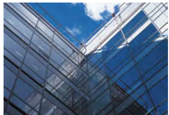
MAYFAIR PLACE London, UK / 2000 EPR Architects
