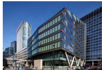
MOOR PLACE London, UK / 2014 Arch. HKR Architects
