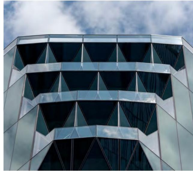
The curves are composed of five panes tridimensional curtain wall units. Each unit has a base of 8'x8' for a typical height of 16' with four triangular panes surrounding a rhomboidal central pane. This system enables the signature "solar carving" at the North-West and South-East corners of the building elevations, creating an extremely original and iconic aesthetic effect.
