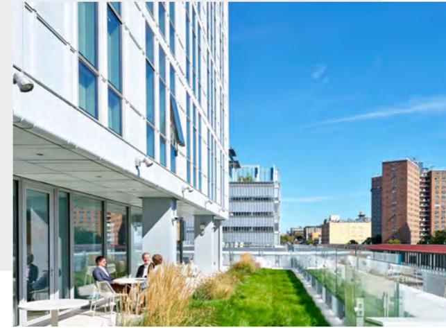
Focchi scope of work was including the design-assist, engineering, fabrication of unitized curtain walls, custom storefronts, and an extensive Glass Fiber Reinforced Concrete (GFRC) rainscreen system.
