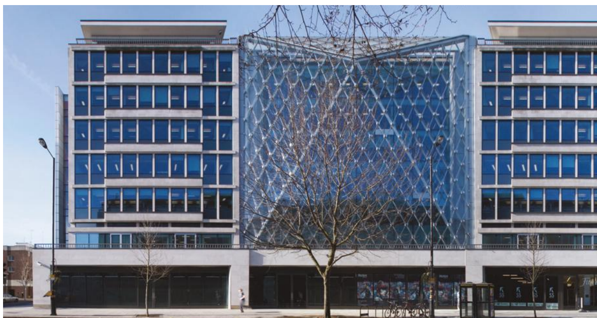
55 Baker Street, London - Zander Olsen, Make Architects
