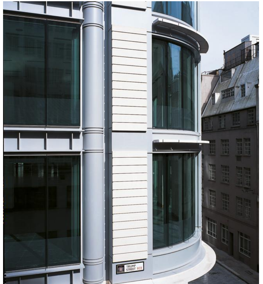
▲ Curved Main Curtain Walling
