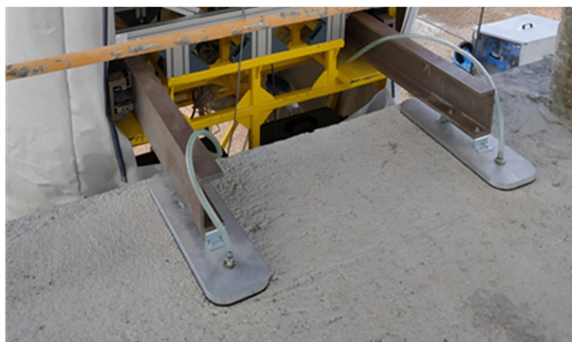
Figure 8. Stabilizer attaching the robot platform to the concrete slab (photo: José David Jiménez-Vicaría).
