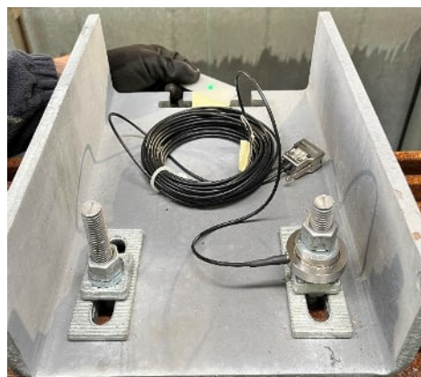
Figure 14. Façade bracket with force washer installation.
