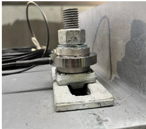
Figure 13. Zoom on the force washer installed on the bracket's bolt.
