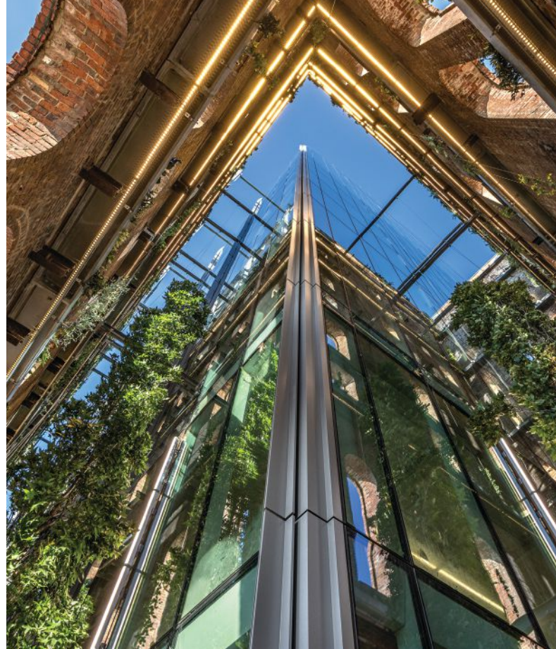
A 10-12 foot gap between the old and new structures creates a space for biophilic design, connecting the outdoors and indoors.
