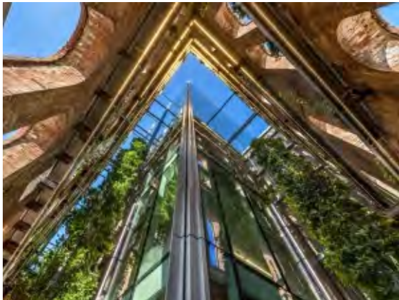
The glass office building took shape inside the original structure. Image by Max Touhey, courtesy of PAU
